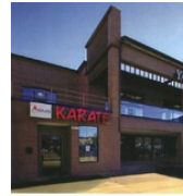
View of lower-level entrance to new location
